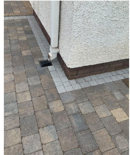
Show the drainage (gullies, drainage channels etc)
