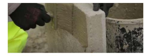
Blocks should be placed by hand onto the prepared laying course and tapped into place using a paviours maul.
