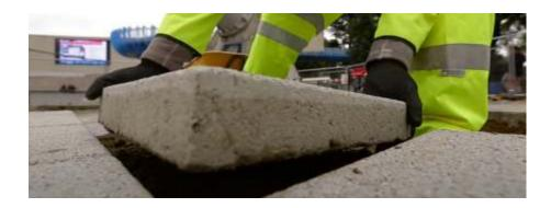
The laying course material should rise upwards into the joint. Minor adjustments necessary to maintain the laying pattern should now be made. A laying method which maintains an open laying face, should be used.
