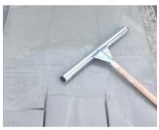
Use a squeegee to move the slurry over the surface and ensure that all open joints are adequately filled.
