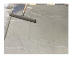
Joints should finish 3 mm below the pavement surface. Completely soak the entire area to be jointed with clean water and spread the mortar slurry over the area.
