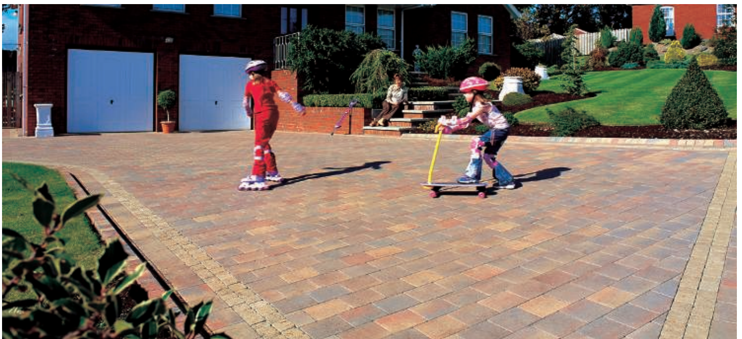
Image 7 - Driveway with blocks correctly blended.
