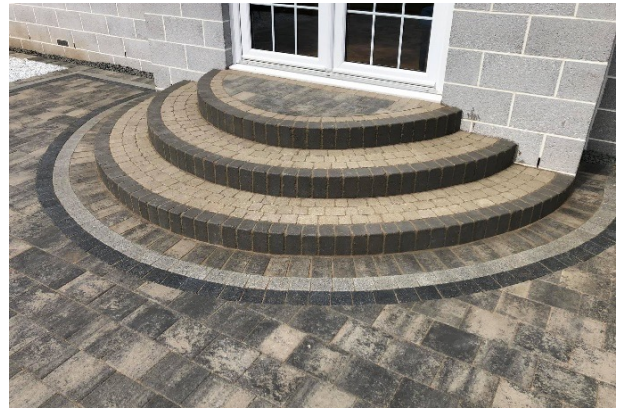
Multiple Semi-circular steps with block paving infill
