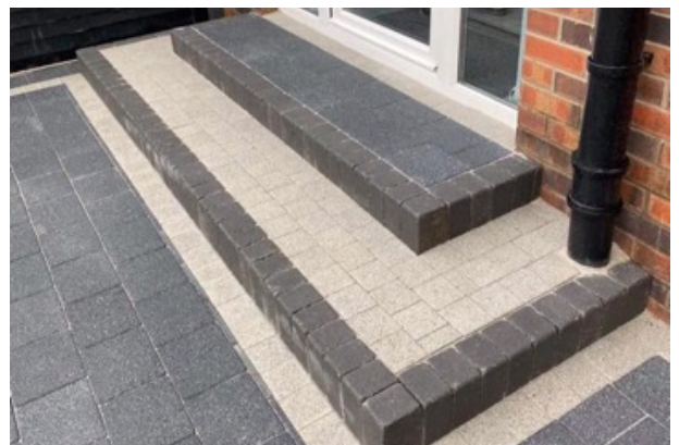
Multiple Rectangular Steps with block paving infill
