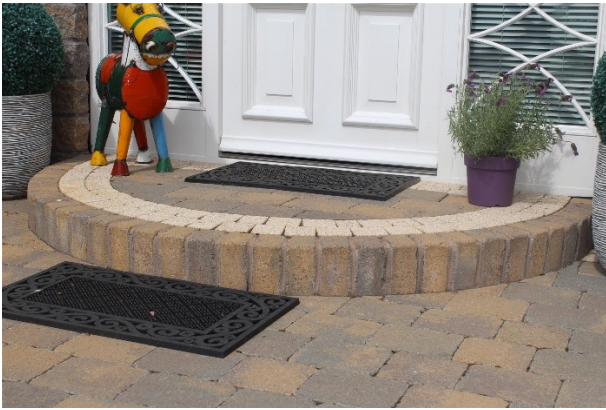
Single Semi-circular step with block paving infill
