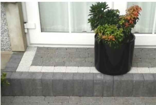
Single Rectangular Step with block paving infill
