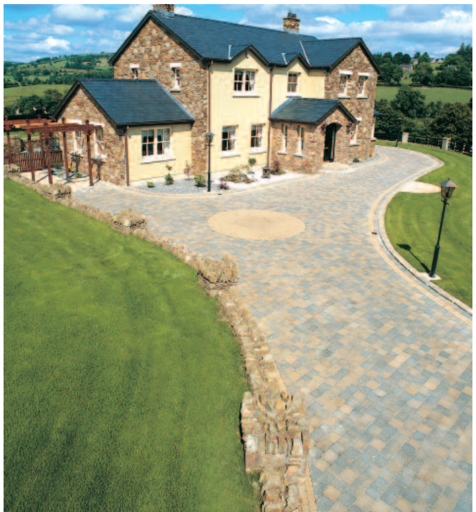
Premier Design Service – Not only did the customer benefit from a beautifully paved driveway with a uniquely-styled boundary wall, they also created double family patio areas with steps and circle features for their own private use.
