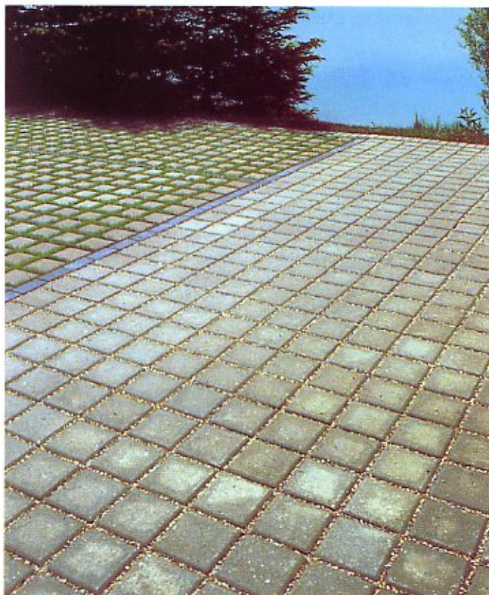
ABOVE The new Rima block which allows drainage or grass growth
